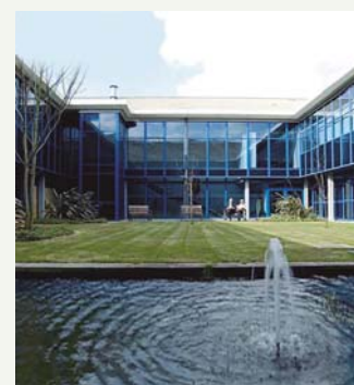
NHS Canford house clinic, Bournemouth, UK. VRF
